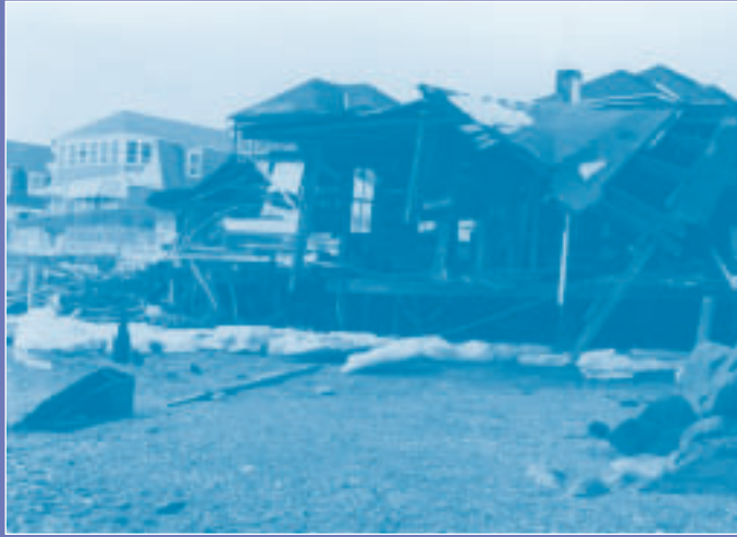
Coastal damage from the storm in 1978.
