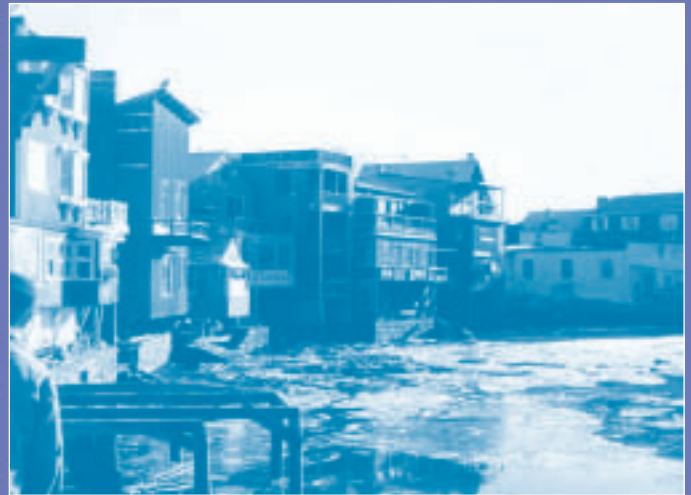
1978 storm damage to Rockport Harbor.
