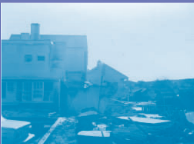
Destruction in Rockport from the storm of 1978.
